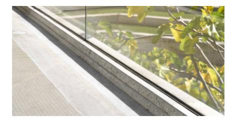
groovEe<sup>™</sup> is the latest innovation from EeStairs continued drive to deliver major advances in stair and balustrade systems. groovEe<sup>™</sup> accelerates the production and delivery of stylish, highly durable, cost-saving glass balustrades for concrete balconies.
